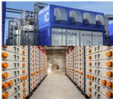
(Flow battery / Lithium Ion)
